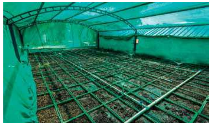
Figure 1(b): Inside view of Bio-filter Basin
