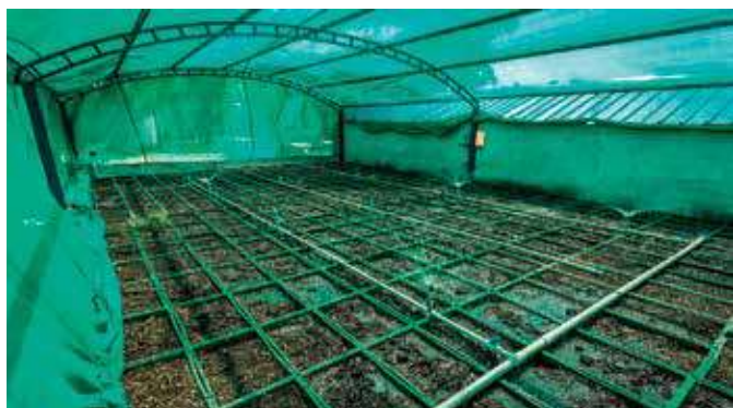
Figure 3(a) Civil based Bio-filter (for larger capacity) and
